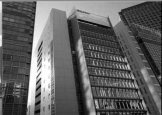
Figure 2. Nikken Tokyo Building, Japan, 2003.
